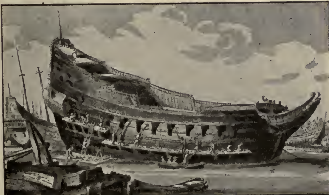
DUTCH EAST INDIAN WARSHIP OF THE SEVENTEENTH CENTURY UNDERGOING REPAIR
