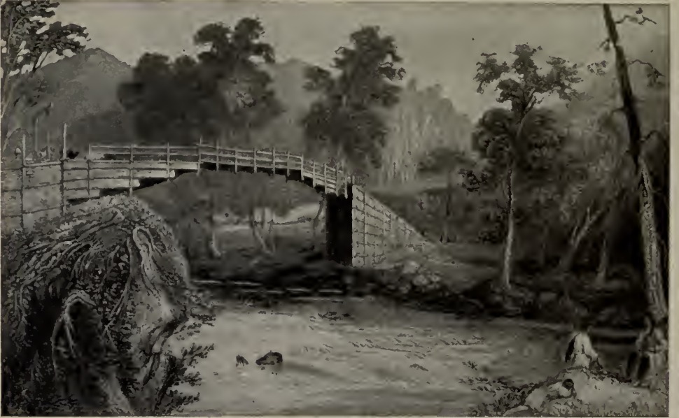
WOODEN BRIDGE AT BHURKOTE IN THE HIMALAYAS
